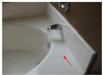
View of master bathroom tub faucet not extending past the lip/edge of the tub.
