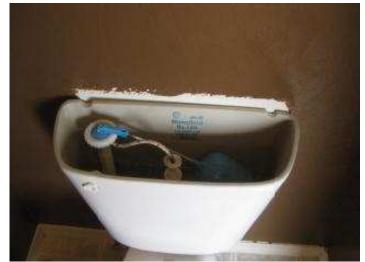
View of master bathroom toilet with broken clapper handle and missing tank cover.
