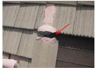
View of slipped tile and cracked mortar cap next to asphalt shingle roof to AC/Heat pump.
