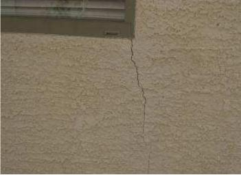
View of typical cracking in stucco at exterior window to NW bedroom.
