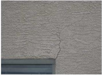
View of cracking in stucco at south facing window to master bedroom.
