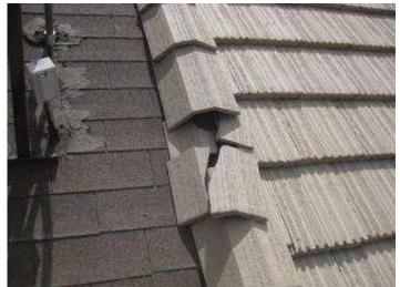
View of cracked tile at west facing roof slope next to asphalt shingle roof to AC/Heat pump.
