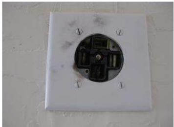
View evidence of charring at open faced 30 amp electrical receptacle for dryer.
