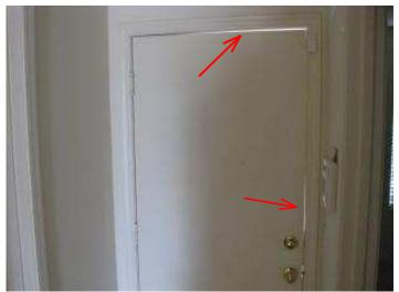
View of garage service door to home not fully self-closing and latching.
